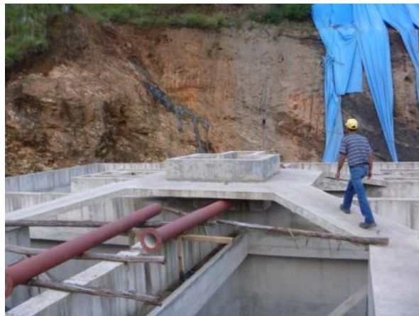
Figura 1.20 – Reator UASB inacabado
