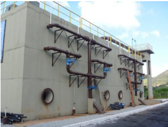
Figura 1.14 – Reator UASB
