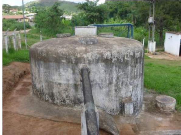
Figura 1.7 – Reator UASB
