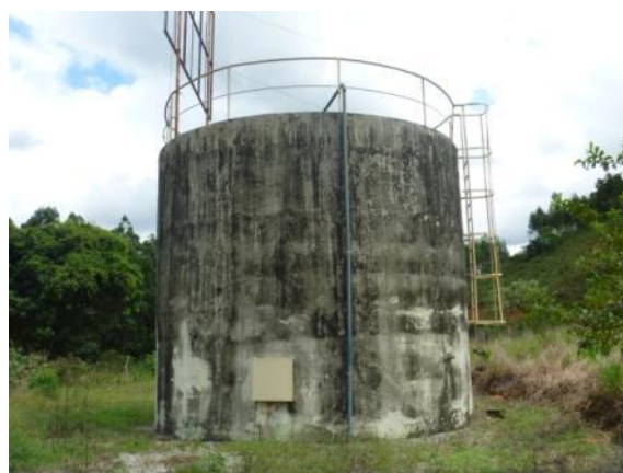
Figura 1.11 – Reator UASB
