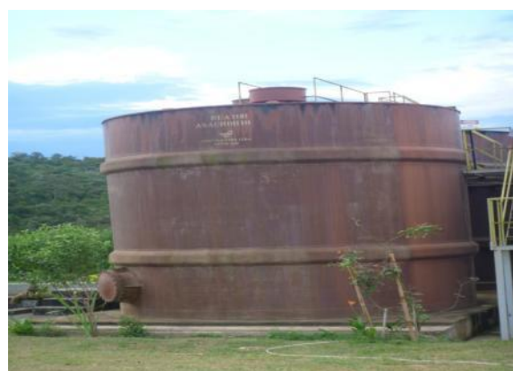
Figura 1.7 – Reator Anaeróbio
